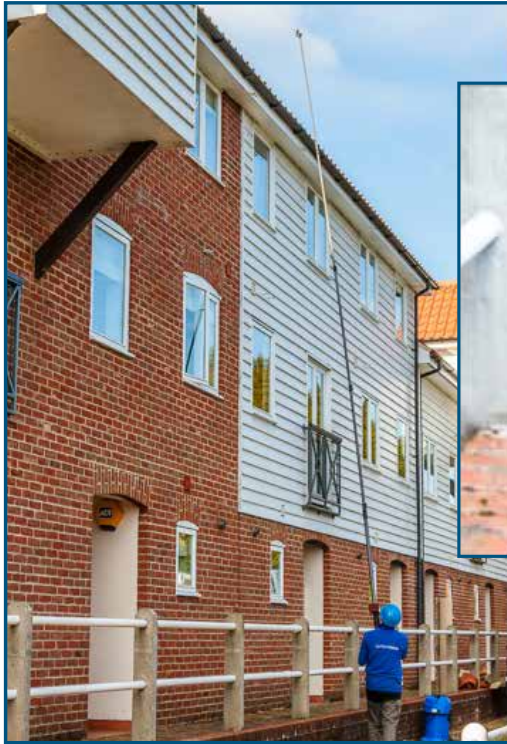
Camera survey conducted in order to provide quote.
